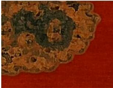
Water Soluble Corrosion
